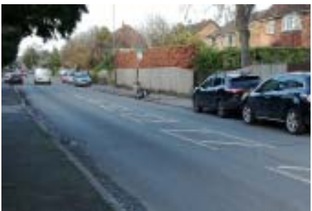
Parking on pavements on A4094
